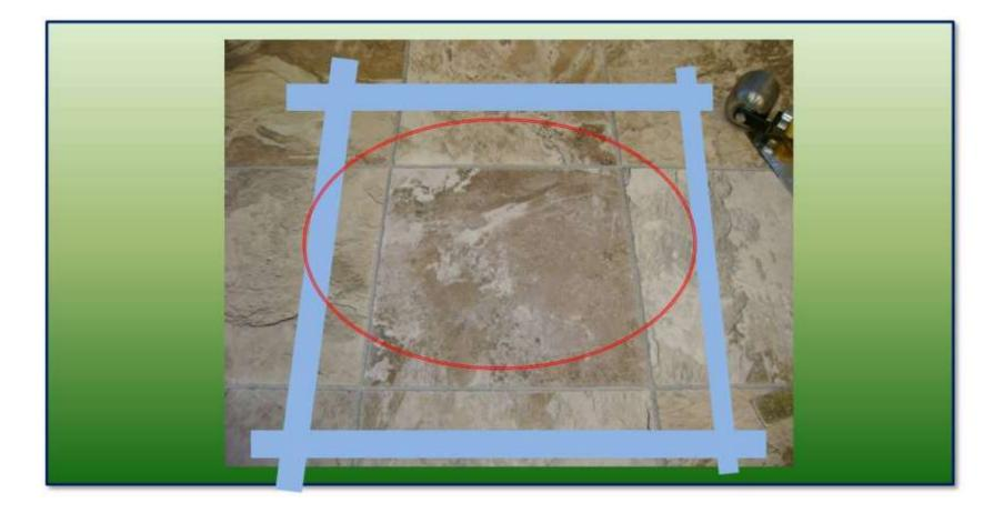
•The serviced area should appear virtually invisible from a standing position when properly completed. Remove the painter tape within 2 hours of completion.
