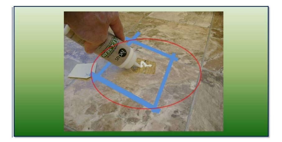
•Apply the Flex-Seam in the opening & under the vinyl the length of a minimum of 2" and on the edges in preparation of inserting the graph.
