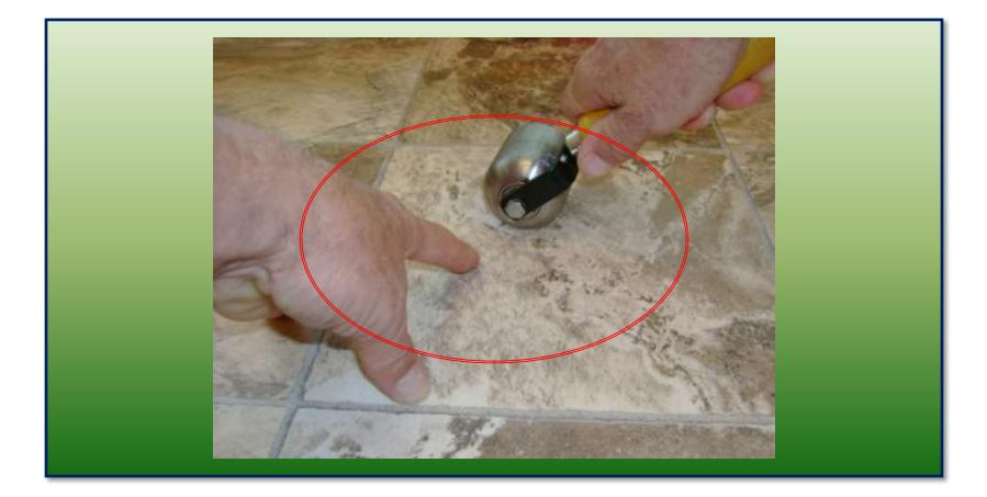
•Using a hand roller, roll the damaged area to remove excess adhesive and flatten the wrinkles
