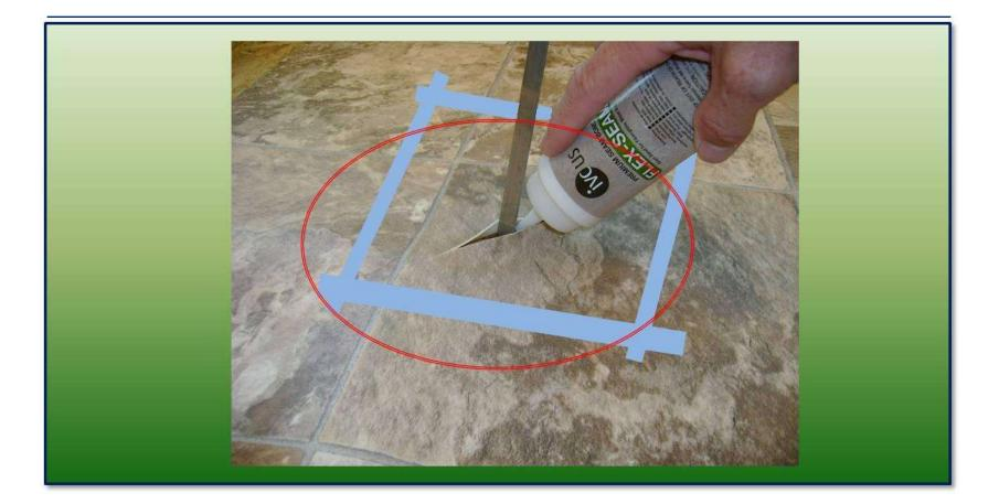
•Apply a small amount of Flex-Seam under and on the edge of the sliced area.
