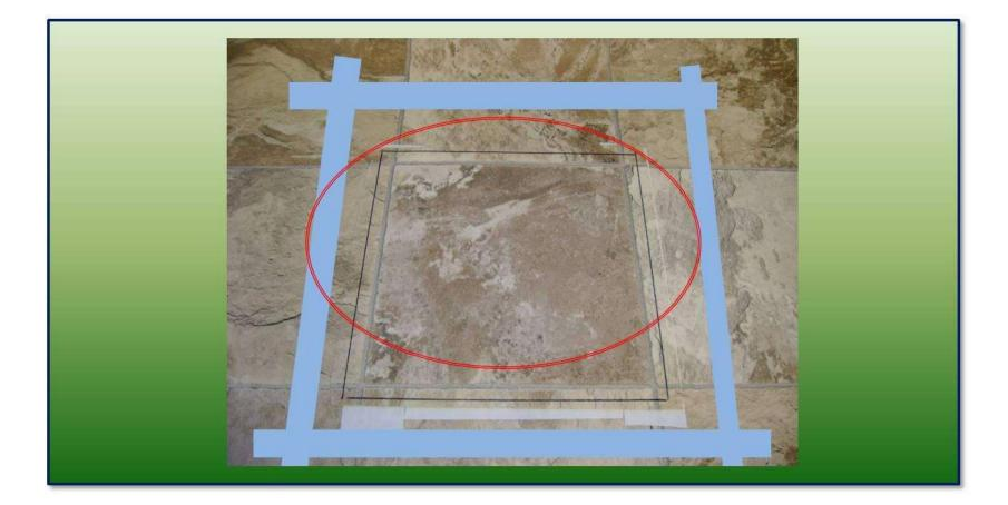
•Place the replacement section of vinyl on top of the double face tape properly aligning the pattern
