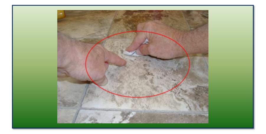
•Once the damaged area is together clean the excess Flex-Seam off the surface using a clean cloth dampened with water
