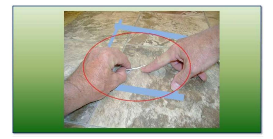
•Gently work the damaged area assuring the slice has been fully coated with the seam sealer.
