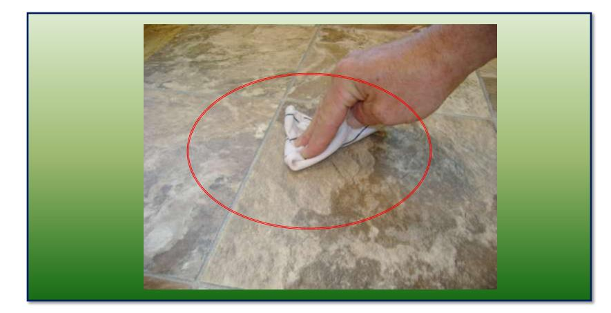
•The damaged area should be flat and ready for cleaning with a damp cloth followed by a clean dry cloth
