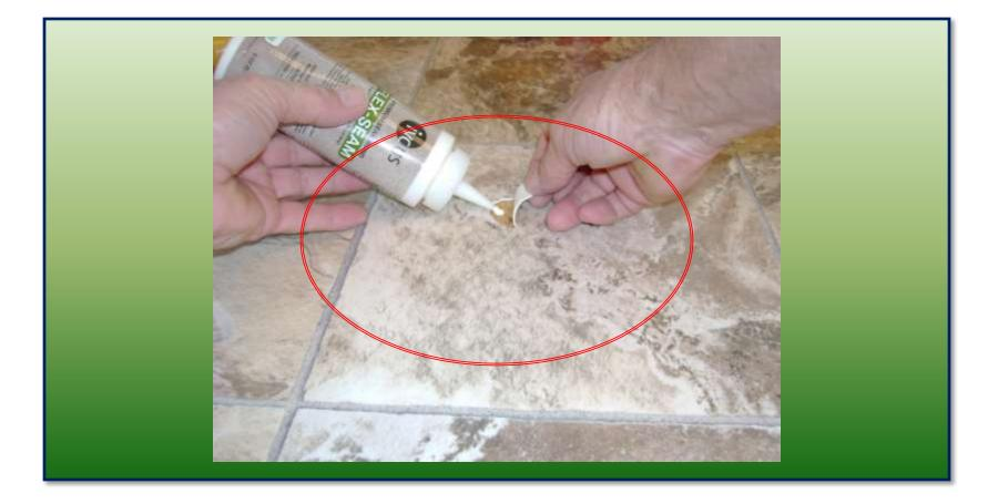
•Apply a small amount of Flex-Seam under the Rip/Tear and along the edges of the Rip/Tear
