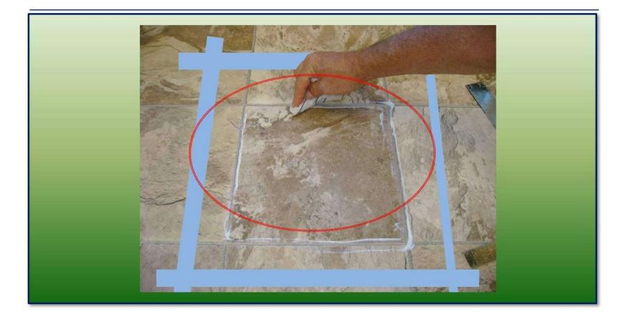
•Using a clean cloth dampened with water remove the excess Flex-Seam forced to the top.
