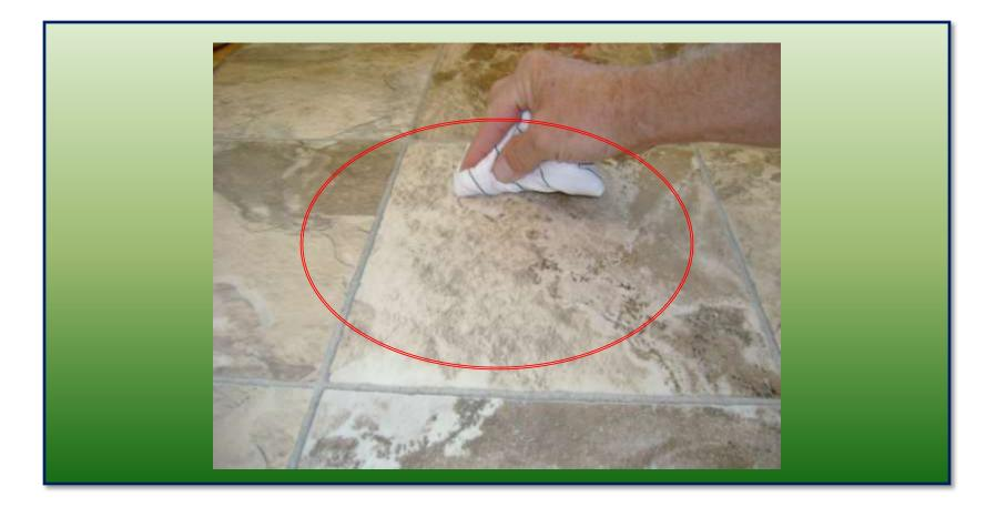
•The damaged area should be flat and ready for cleaning with a damp cloth followed by a clean dry cloth
