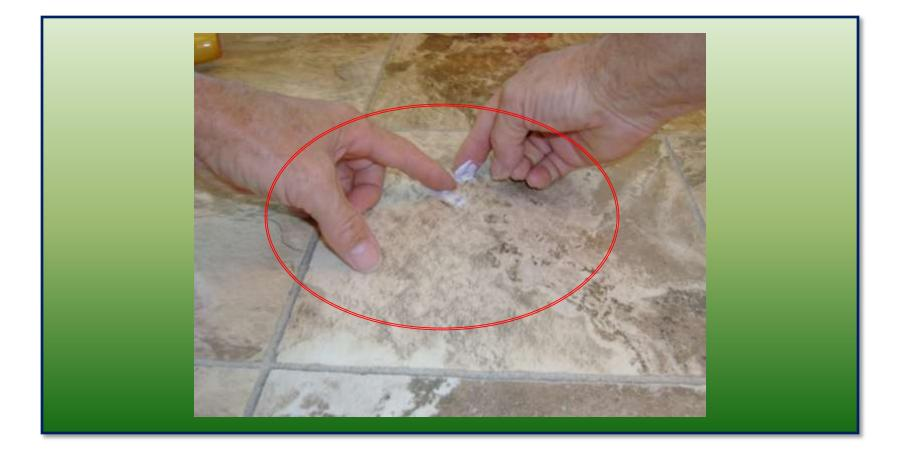
Gently work the damaged area into the surrounding area being sure all edges are properly aligned
