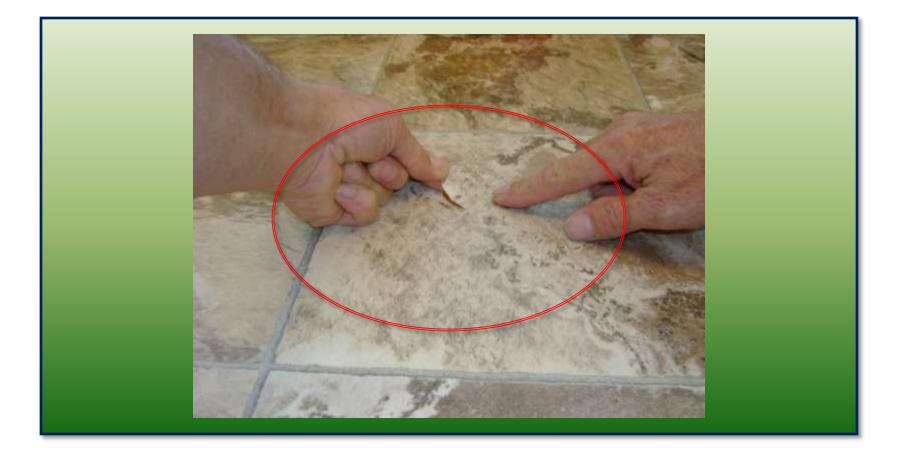
•Gently open the damaged area applying light pressure to remove the wrinkles
