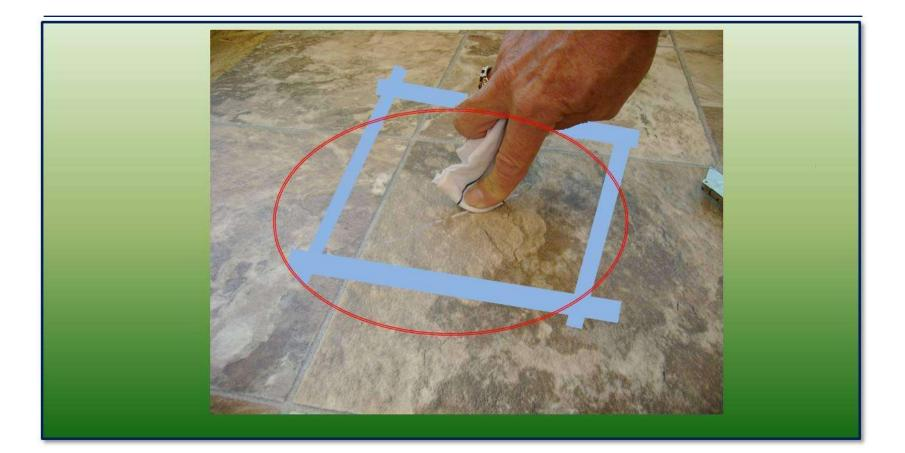
•Once the damaged area is together clean the excess Flex-Seam off the edges of the vinyl using a cloth dampened with water
