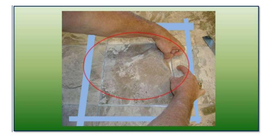
•Place the replacement section of vinyl into the opening (remember to match the Identification marks)
