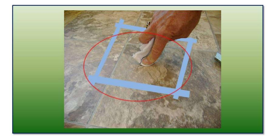
•The damaged area should be flat and ready for cleaning with a damp cloth
