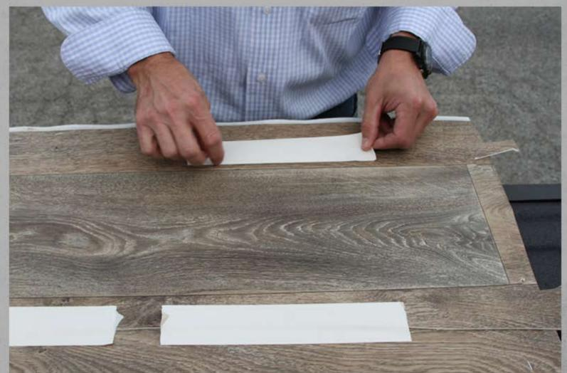
• Cuts should be made in grout or plank lines or areas where the flooring pattern will disguise patch edges.
