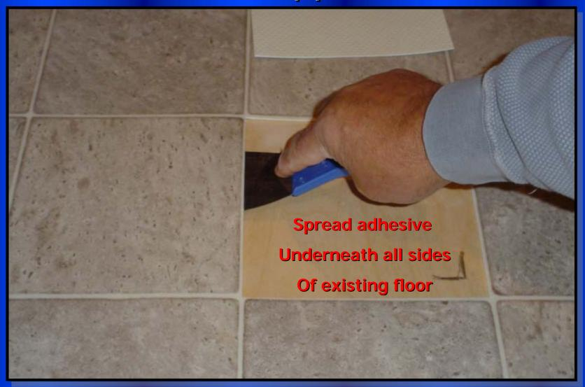
With a notched spreader, surround the cut area beneath the remaining floor with a 3-4 inch band of acrylic emulsion adhesive.
