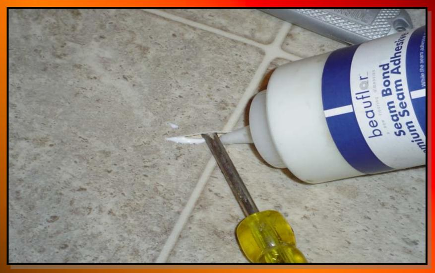
Using a clean screwdriver hold the edge of the material apart and apply seam bond adhesive.
