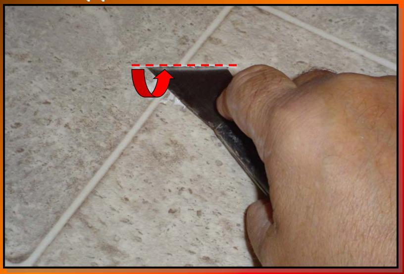
With a small putty knife, work acrylic emulsion flooring adhesive under the material as far as possible in all directions.
