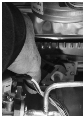
Remove gas line 19mm or 3/4" wrench
