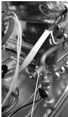
Input Thermistor
