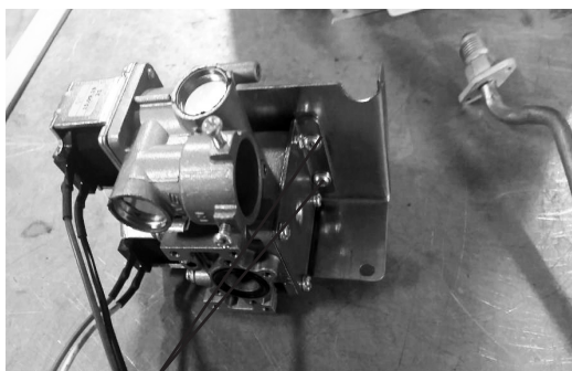
Gas Valve Bracket Screws
