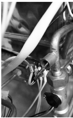
Input Thermistor
