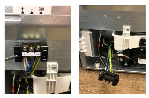
Remove 2 philips screws holding power terminal on the back of the refer in place.
