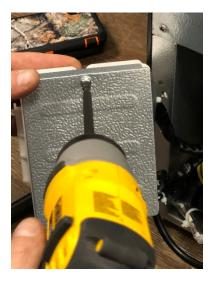
Remove the Philips screw that holds the cover in place. Once that screw is removed the cover will pop off of the box.
