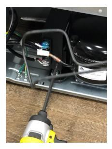
Once you have the pan removed, remove the Philips retaining screw holding the compressor board in place.
